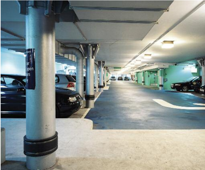
Bristol Municipal Car Park
